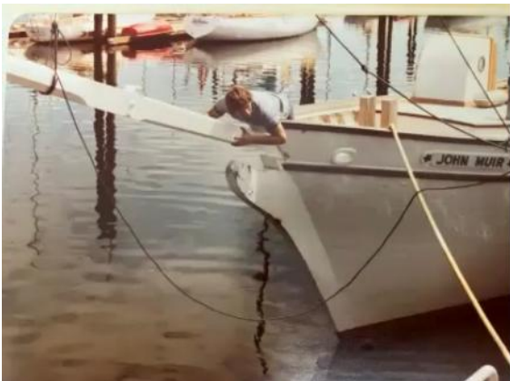
Aligning the Bowsprit
